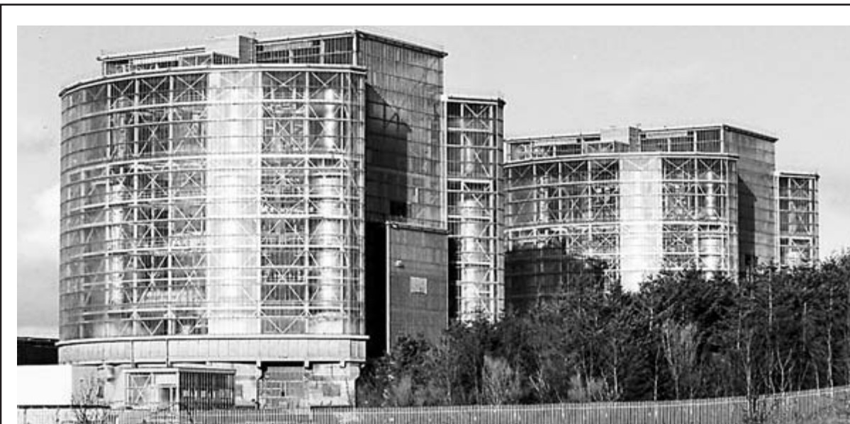
HOME AND AWAY: Hunterston B and, far right, Canada's Bruce Power plant run by Duncan Hawthorne, inset
